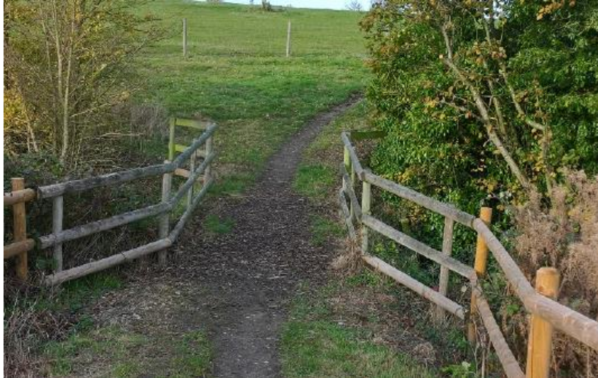
Proposed route over existing bridge carrying footpath CALW40
