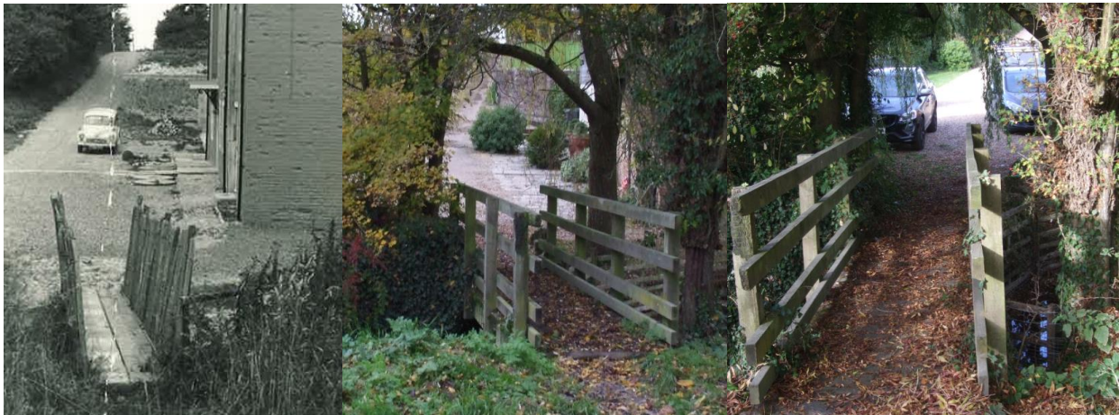
c.1968 (temporary bridge in place)
